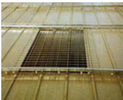
Figure 4.8: (a) Galvanised mesh reinforcement between sheets of twin skinned rooflight and (b) guard-rail fitted over a rooflight.
