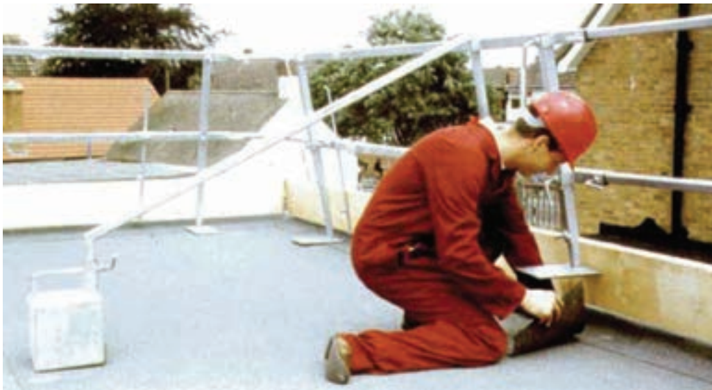
Figure 8.5: Temporary flat roof edge protection. Adjustable supports enable work to progress with protection in place.
