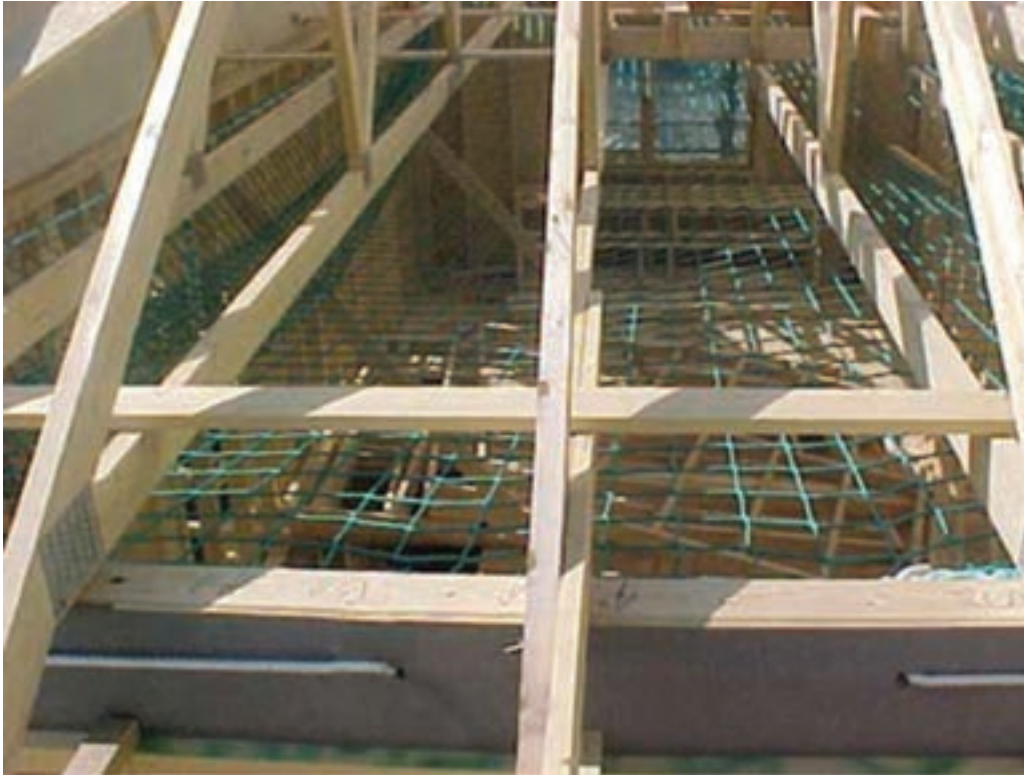
Figure 8.3: Safety nets used to give collective protection in the erection of housing roofs
