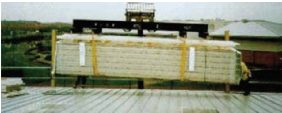
Figure 9.2(a): Delivery of sheets to roof level onto the completed load-bearing section and behind the leading edge. (Note the rooflights include mesh protection rendering the assembly non-fragile.)
