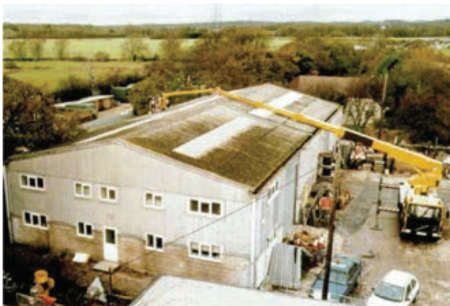
Figure 13.1: Powered access for the inspection of a large fragile roof.
