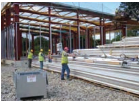
Figure 12.1: Mechanical aids for rotating and lifting cladding sheets.
