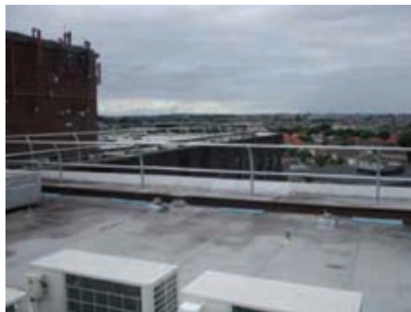
Figure 4.5: Permanent guard-rails retrofitted during refurbishment work. Similar protection can be included during initial designs.
