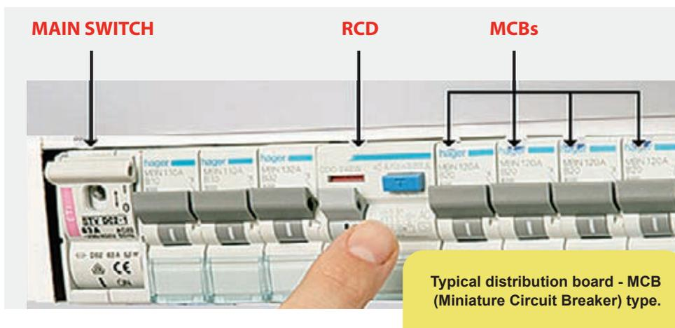
Check that your RCD is working correctly by pressing the test button marked 'T' or 'Test'. Remember this will cut the power to all socket outlets so make sure no essential work is being done at the time.
